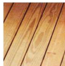
Treated Decking Boards on Porch Floor
