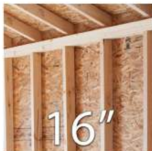
16" on-center Walls, Roof, & Floor Joists
