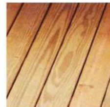
Treated Decking Boards on Porch Floor
