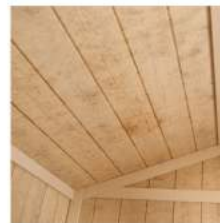
Paneling on Walls and Ceiling
