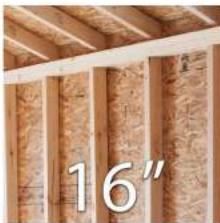
16" on-center Walls, Roof, & Floor Joists
