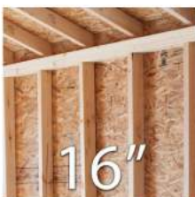
16" on-center Walls, Roof, & Floor Joists
