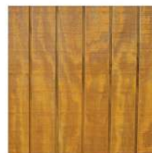
Sealed w/ Exterior Grade Stain
