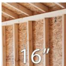
16" on-center Walls, Roof, & Floor Joists
